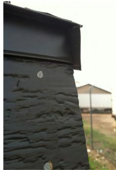
Make sure to fasten the fascia every 24" o.c. maximum. Use Diamond Kote® touch-up paint on all face nails.
