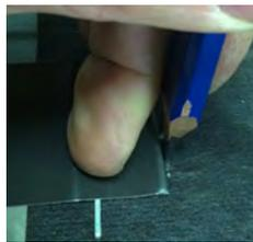
Trim the edge of the metal roof once it is installed on the gable ends or around the corners (for hip roof lines).
