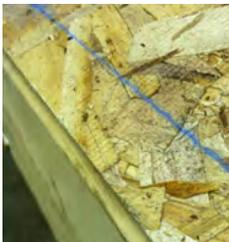
**STEP 2:** While in the same position as Step 1, mark the top edge of the metal roof edge on the roof sheathing.
