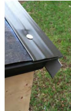
**STEP 8:** While holding it in position, mark the edge of the metal roof edge onto the roof underlayment.
