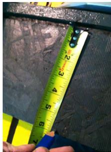
**STEP 13:** Measure and mark the LP® SmartSide® Fascia from Step 12 at the recorded measurement. It is important that this measurement be pulled from the dado as shown. Rip the Fascia to width, and use Diamond Kote® touch-up paint on all cut edges.
