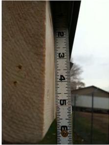
**STEP 12:** Next lift up on the metal roof edge on the eave end and slide your ruler up until it bumps the top of the inside. Record the measurement where the bottom of the sub-fascia ends.
