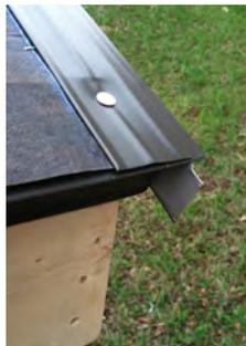
**STEP 14:** Cut the fascia to length and paint all cut edges. Start by installing the Fascia on the eaves. First lift up on the metal roof edge and slip the Fascia behind the metal.
