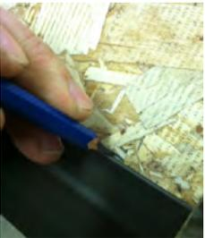
**STEP 1:** Hold the metal roof edge up to the eave edge of the roof line. Keep the top edge of the metal on the plane of the sheathing, slide the metal roof edge up or down the roof until a 5/8" measurement is achieved perpendicularly out from the Fascia to the inside of the bend in the metal roof edge.
