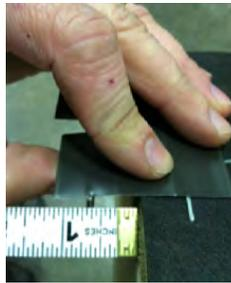
**STEP 4:** Install the metal roof edge by aligning to the chalk line and fasten. Be sure excess material hangs over past the ends of the roof corners, gable or eave intersection.
