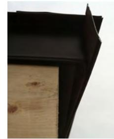
Then slide the metal roof edge in or out from the edge of the roof until 5/8" measurement is achieved from the fascia to the inside of the bend in the metal roof edge. Continue to hold it in this position.
